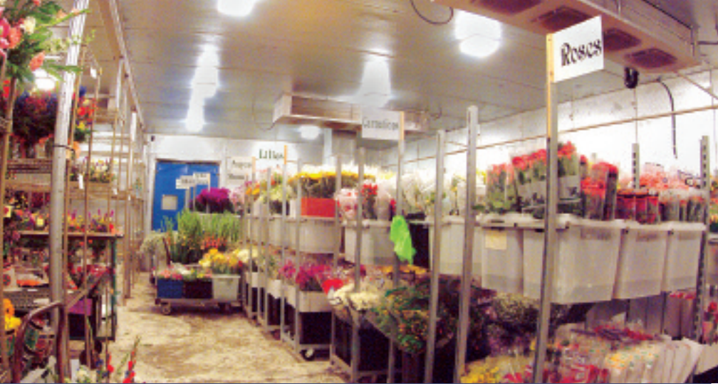
Product stays fresh in Knoll's state-of-the-art cooler that has its own Web site so employees can monitor temperature and humidity levels.
